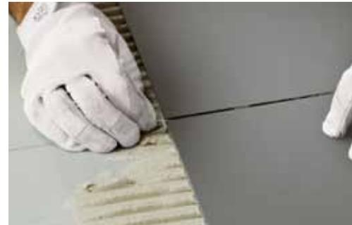
Fit the spacers to create the wished joint: it is recommended to use suckers to aid the exact slab positioning.
