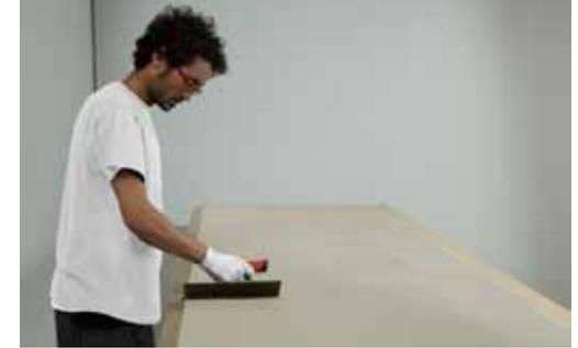
Apply the adhesive with the back-but-tering method in full bed, first on the slab back side and then on the substrate, caring to cover corners and edges, too, and avoid air gaps between substrate and slab. Apply the adhesive gradually only on the surface involved in the application of a slab, to avoid surface film that could jeopardize bonding.
