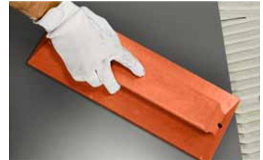
Beat on the surface using a rubber coated squeegee caring to eliminate gaps and air bubbles. Always check the perfect adhesion of corners and edges. Do not walk on the floor during and after the application, respecting the trampling time indicated by the adhesive manufacturer.
