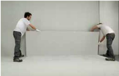
Lay the slab carefully on the long side and, keeping it slightly sloped, lower and apply it and make it adhere on the substrate.
